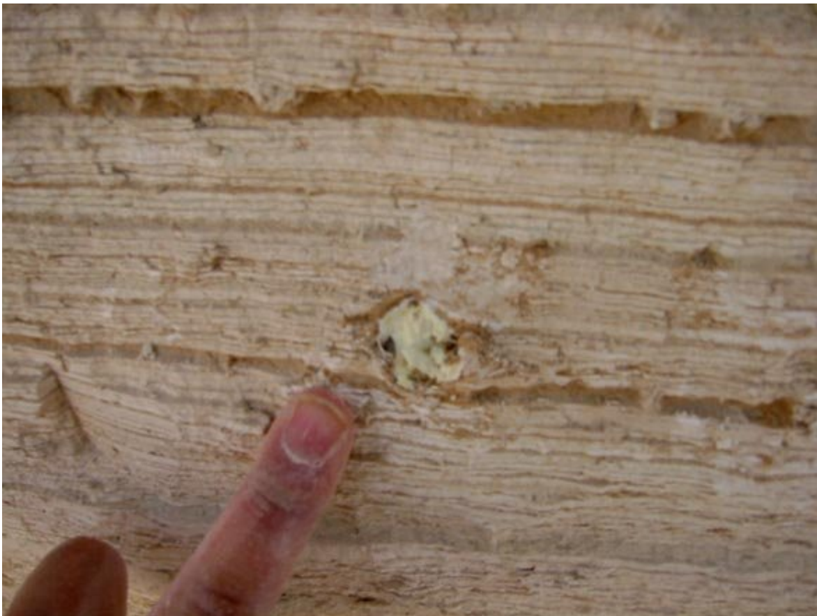
Figure 15 Layering effect caused by ionization
